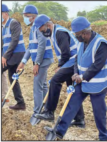
President Grant at the Ground breaking ceremony for housing units at Union Acres, Montego Bay.
